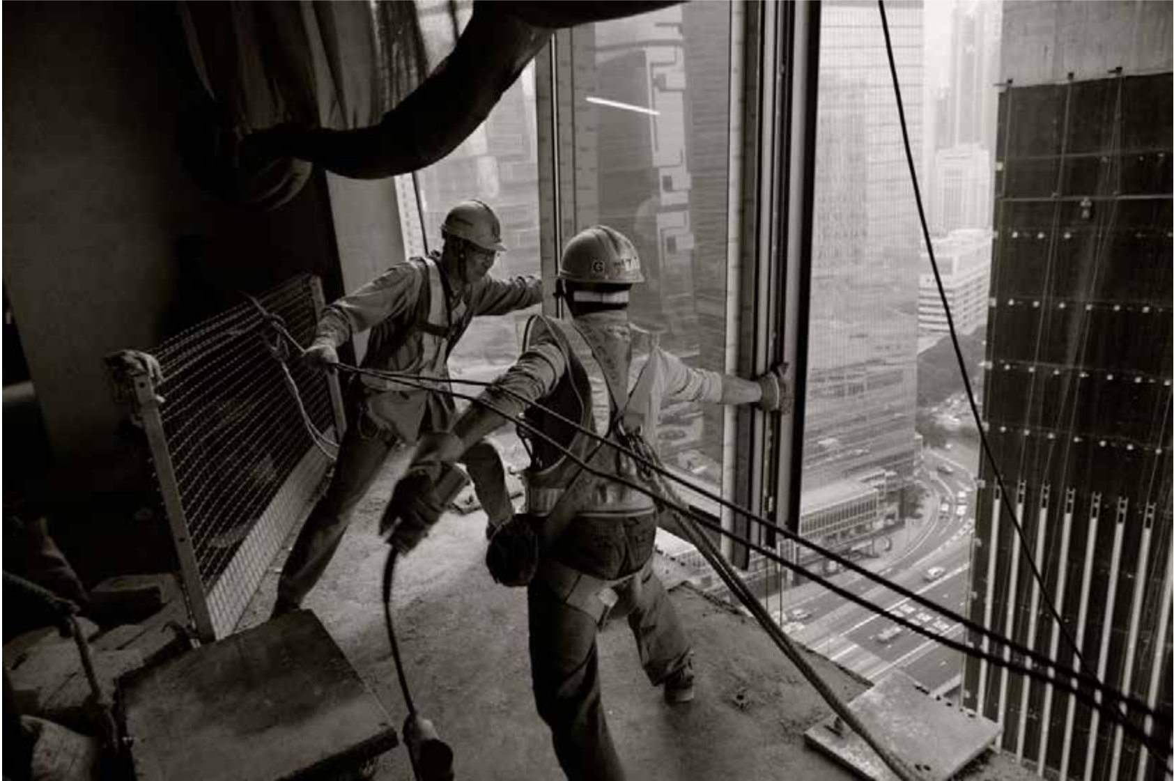
The installation of the CGO curtain wall is a precise and measured process.
